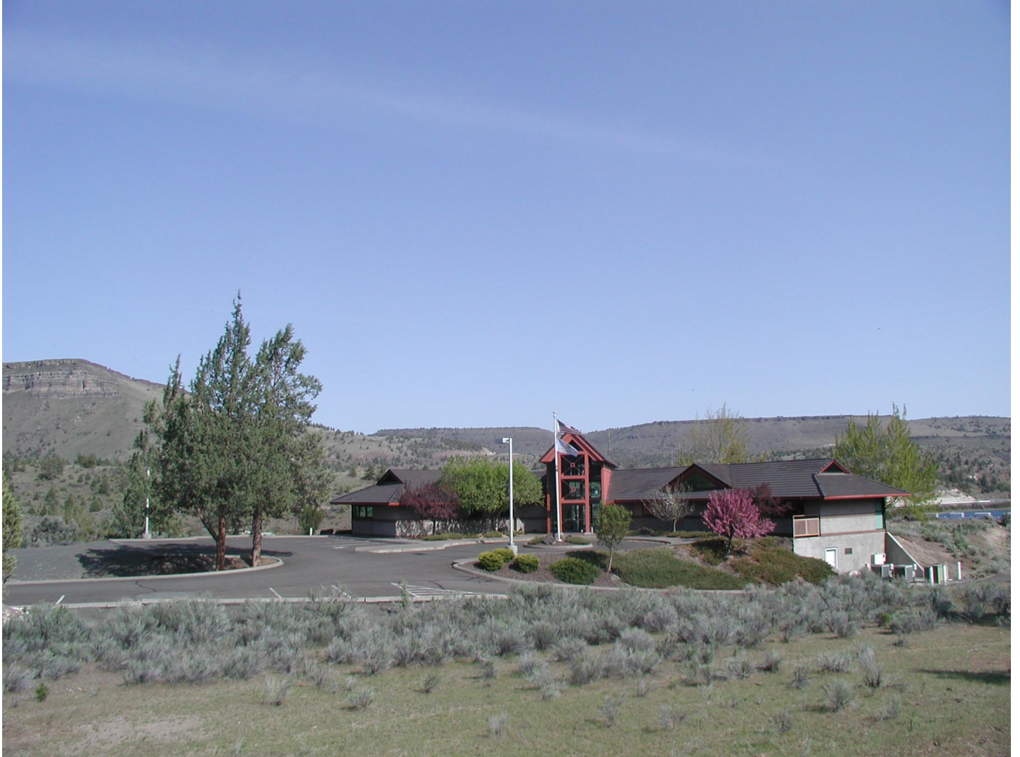
WARM SPRINGS POWER & WATER ENTERPRISES OFFICE BUILDING
