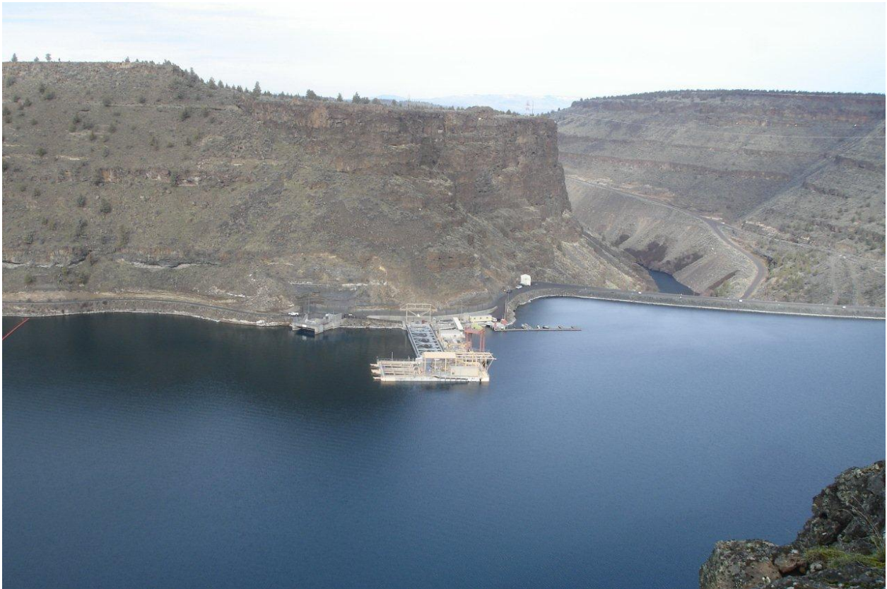
Selective Water Withdrawal Intake for the Round Butte Dam Powerhouse
